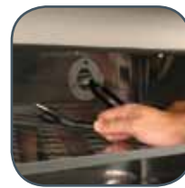
Throughwall Access Port
